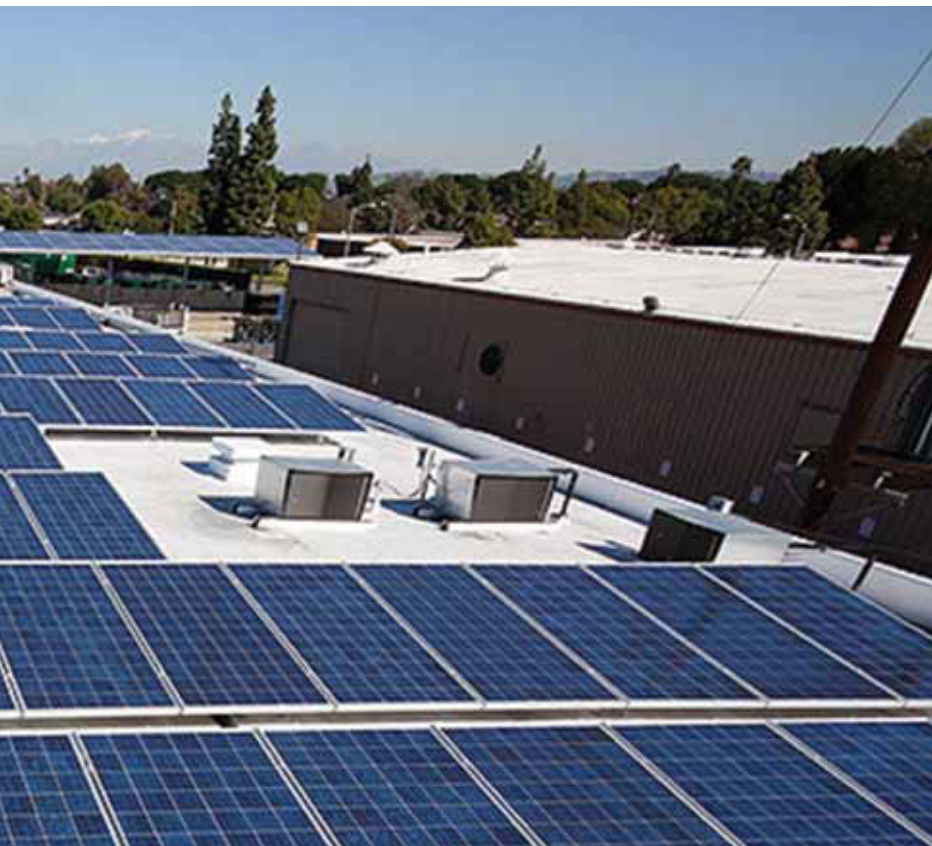
First Class Vending's roof panels collect solar energy, which converts to electric power.
