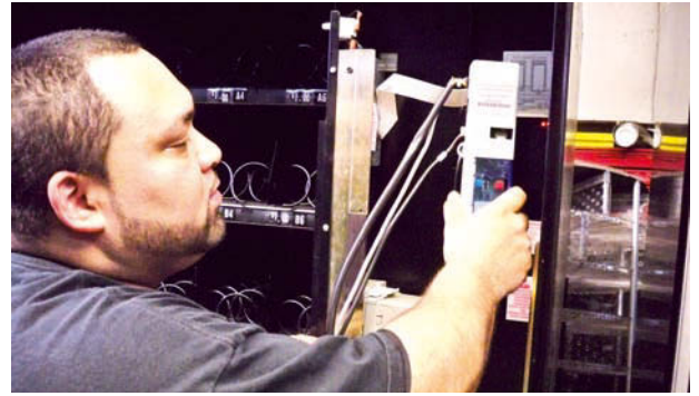
Miguel Filian, maintenance manager at Culinary Ventures Vending, uses the Crane Currenza Navigator to gather data from machines.
